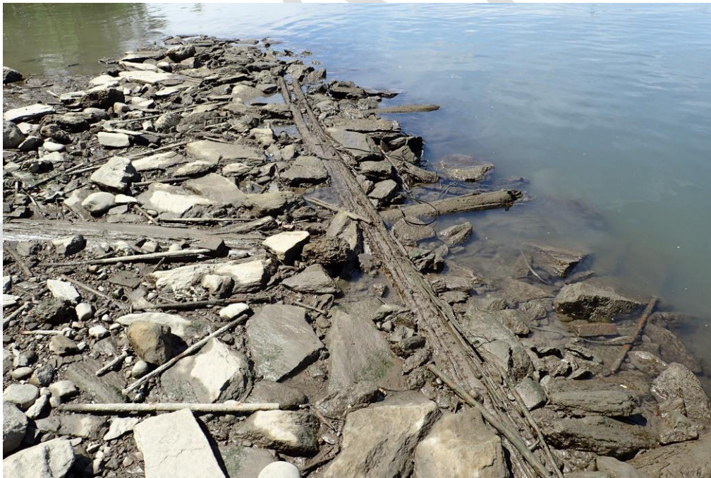
Photo 4: Close up view of timber structure at low tide.
