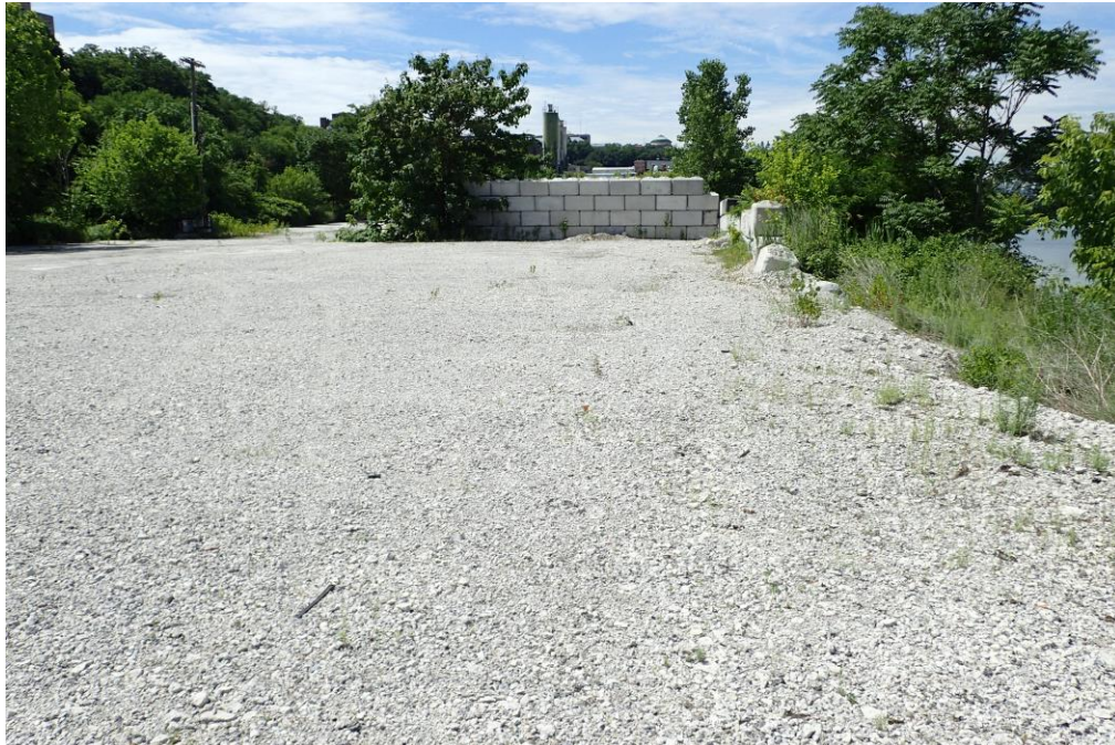
Photo 11: RCA fill on southern third of Lot 3, looking south.
