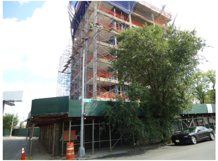
14. Adjacent property to the north-building under construction at intersection of Exterior and E 146 th Streets
