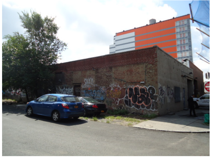
2. Northern elevation of building, facing south
