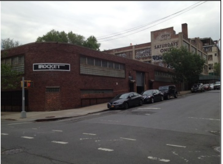
PHOTO 12: Looking at the building located to the east of the project site (across Gerard Ave.) which is occupied by a box company.
