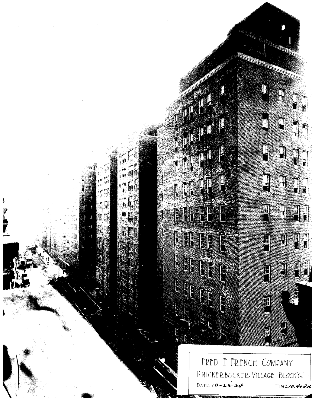
IMAGE 4. View looking east on Monroe Street from Catherine Street—phases of development NYPL, Manuscripts and Archives Division, Fred F. French Companies Records.
