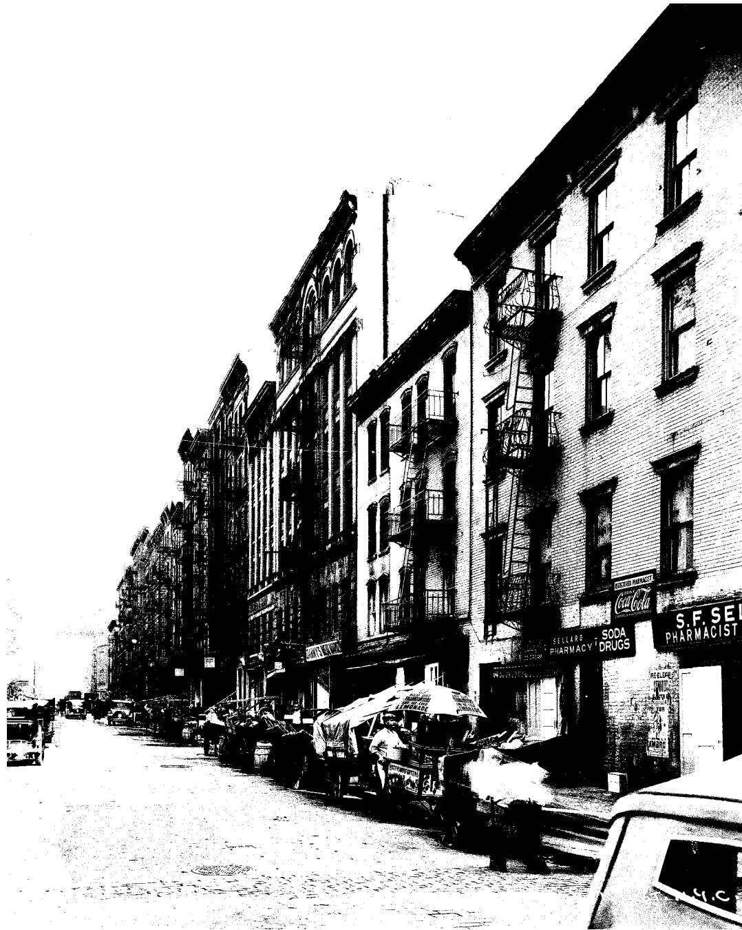
IMAGE 2. View looking east on Monroe Street from Catherine Street—phases of development NYPL, Manuscripts and Archives Division, Fred F. French Companies Records.
