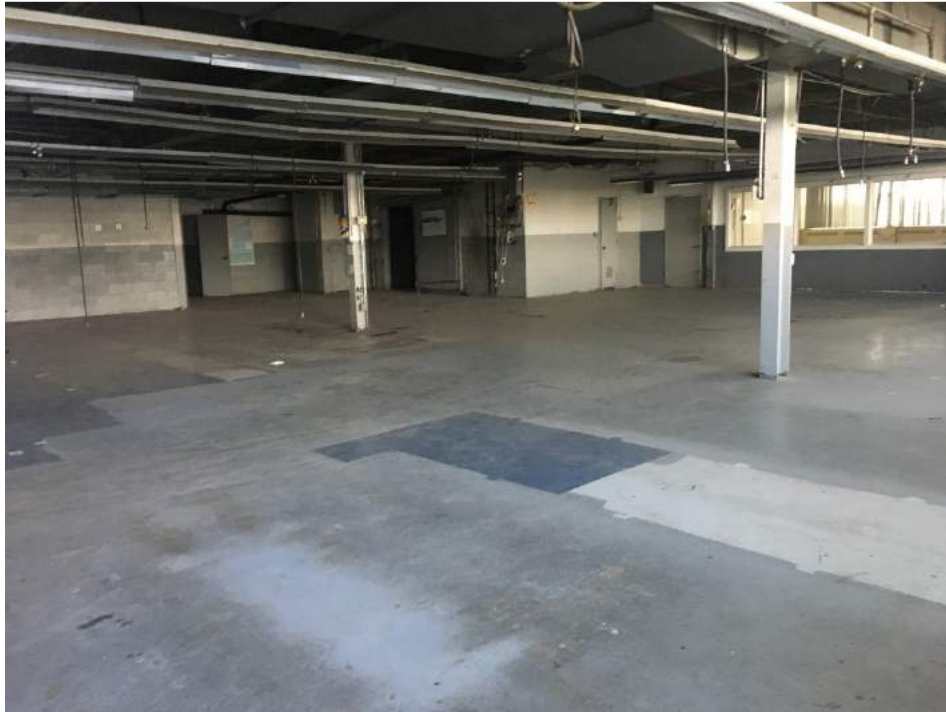
Photo 3: View of the western room on the first floor, facing southwest
