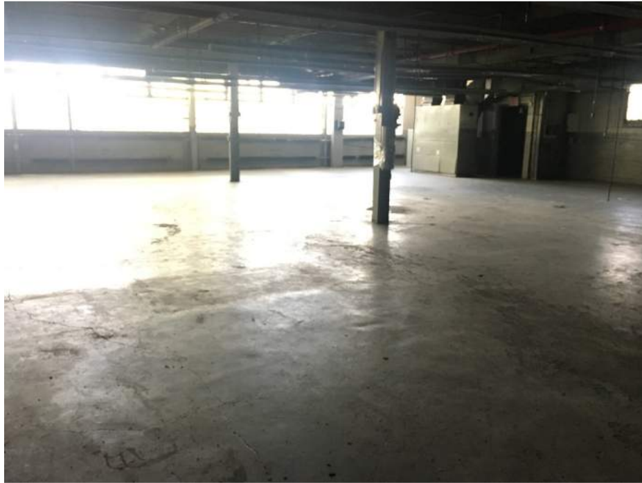
Photo 7: View of the partial cellar, facing northwest
