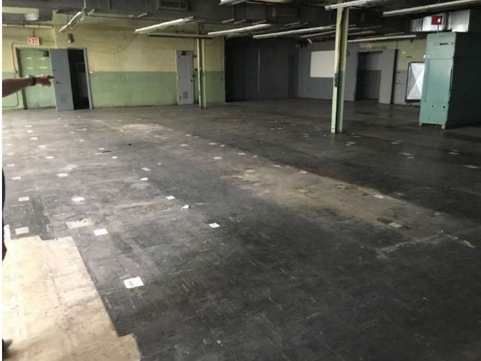
Photo 1: View of the southeastern room on the first floor, facing northwest
