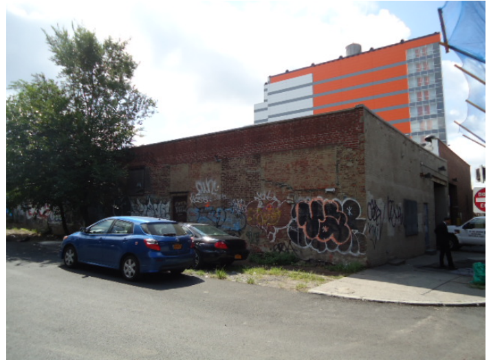
2. Northern elevation of building, facing south
