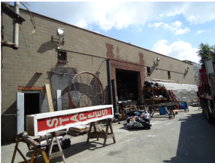
3. Southern elevation of building, facing northeast
